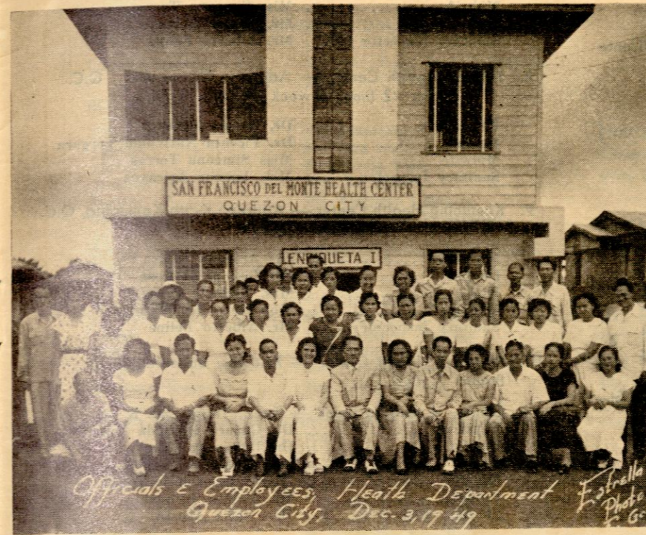
SAN FRANCISCO DEL MONTE HEALTH CENTER (BEFORE)
